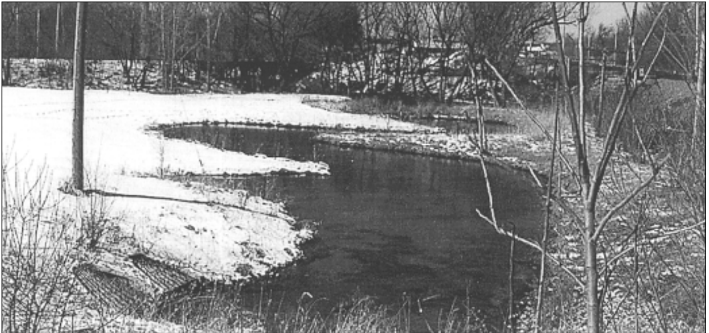
A stormwater Best Management Practice (BMP) is demonstrated by this small recreated wetland which captures stormwater before entering the creek, thereby slowing its velocity and reducing the impact upon the stream.
